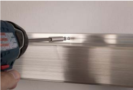
Step 1: Install wall-mount track
